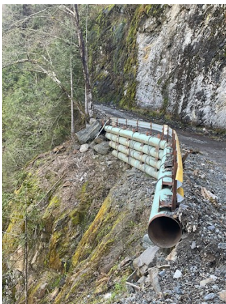
Wall founded on bedrock
