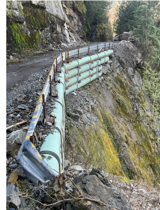
Wall founded on bedrock
